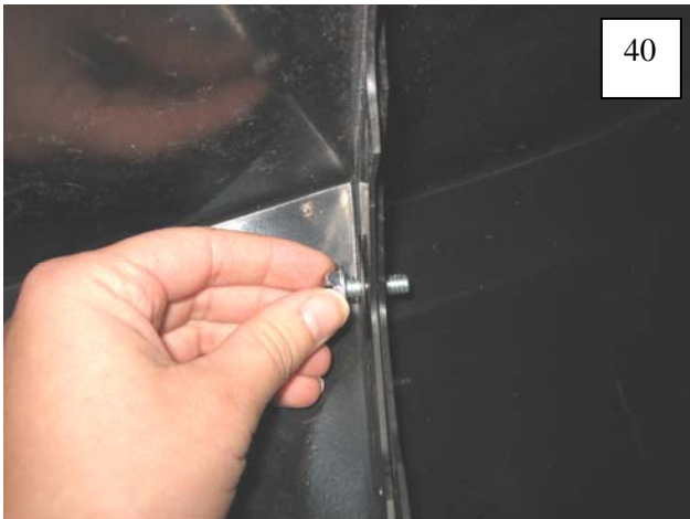
Align the holes in the Rear Main Flare with the holes in the Lower Rear, slide Bolt/Washer assembly through (2 places).
